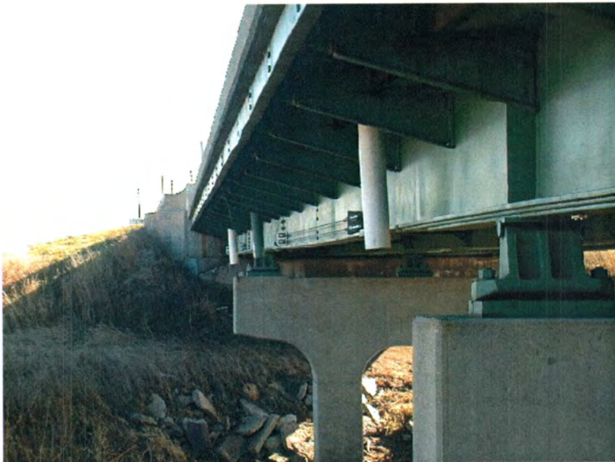
(c) CFRP bars in center span
