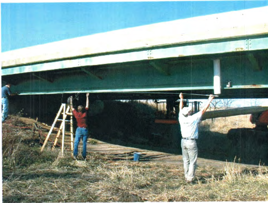
(a) Placement of a CFRP bar
