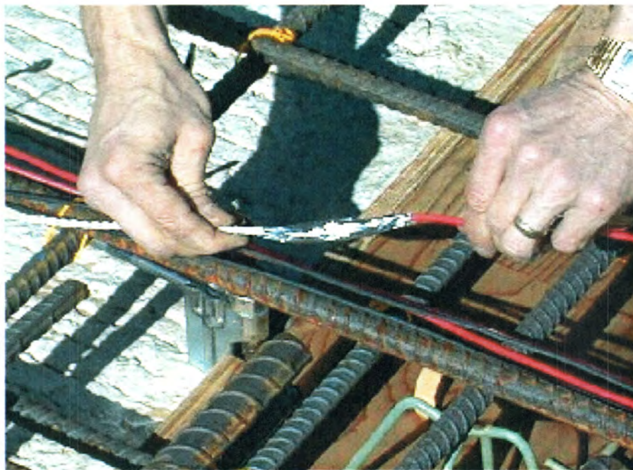
(b) Butt splice protected with butyl rubber underneath aluminum foil tape
