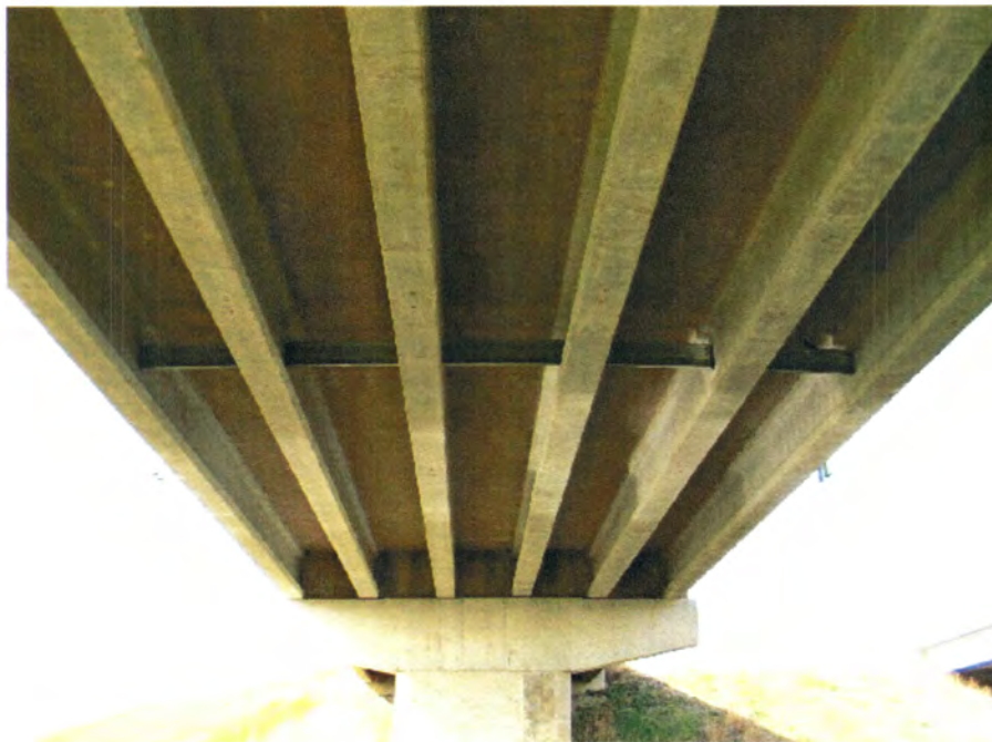
(e) Bottom view (center span and west pier)
