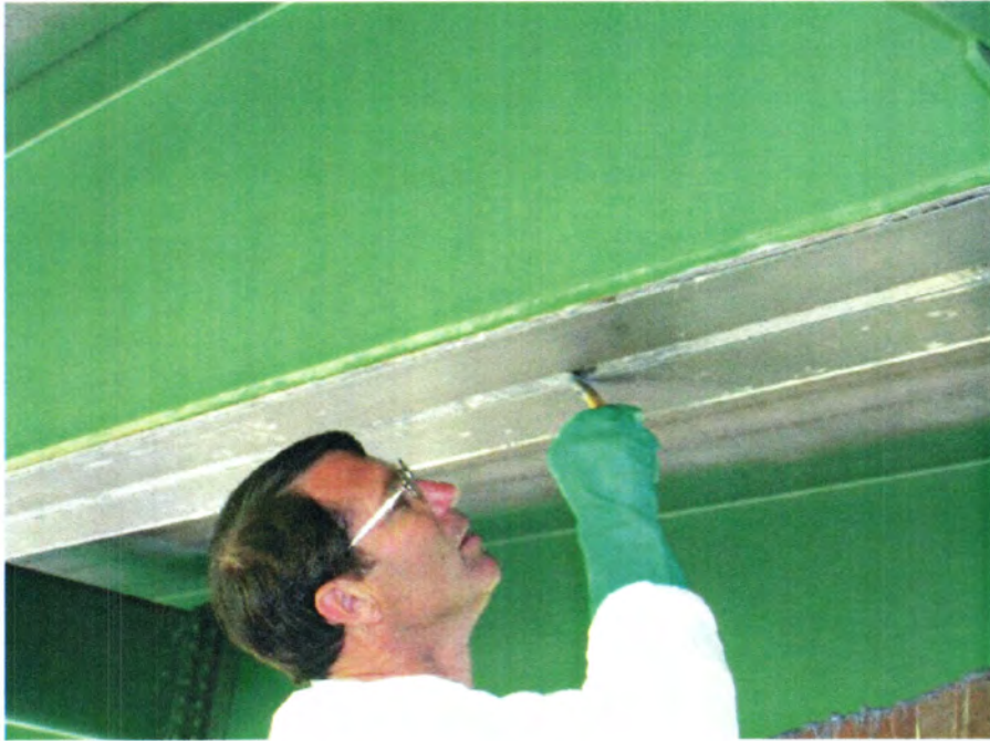
Figure II-20. Removal of excess epoxy.
