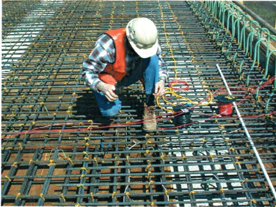
Figure III-12. Extending lead wires for data measurement.
