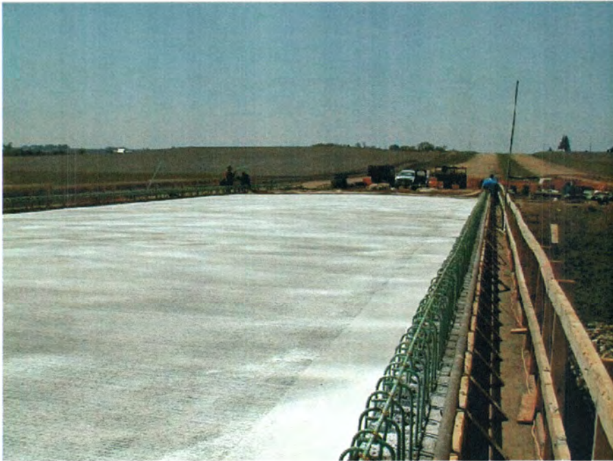
Figure III-6. Concrete placement for bridge deck completed.
