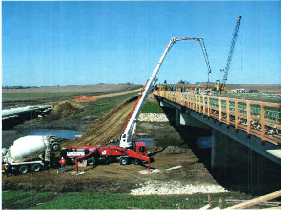
(a) MMFX bridge (looking northwest)
