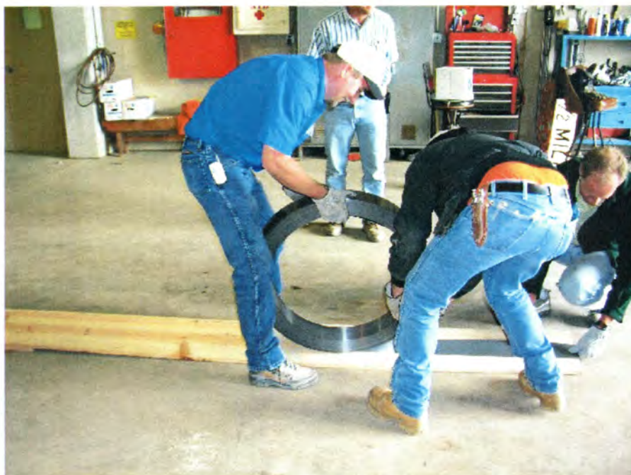
Figure II-3. CFRP plates being unrolled.
