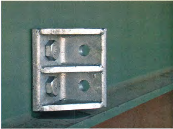
(a) Stiffened steel angle assembly
