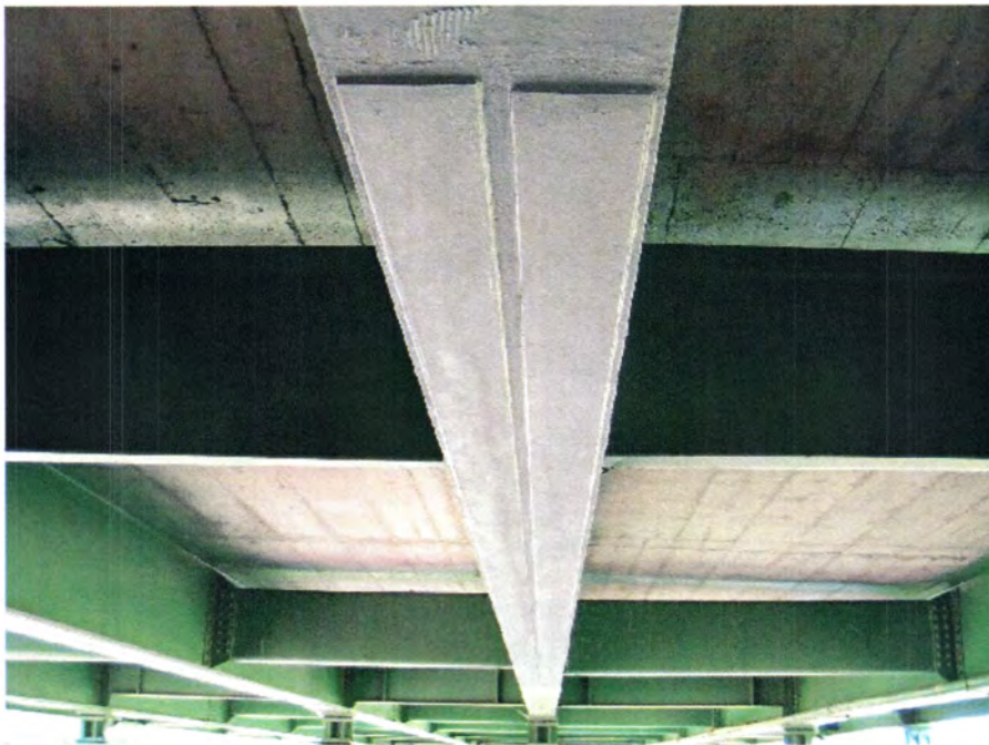
(c) Beam 4 in the east end span
