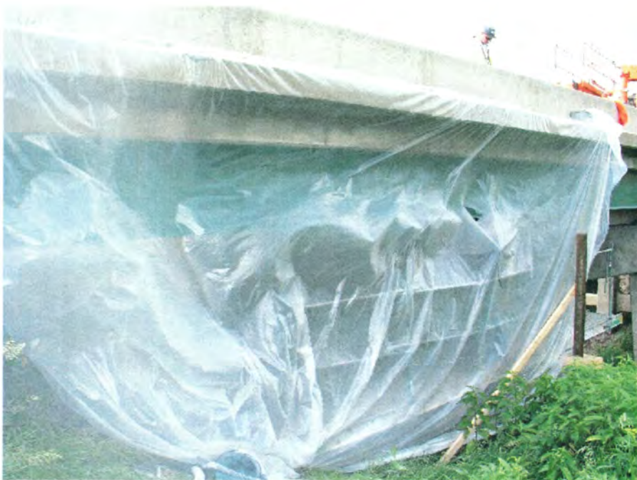
Figure II-10. Work area covered with a layer of vinyl during sandblasting.
