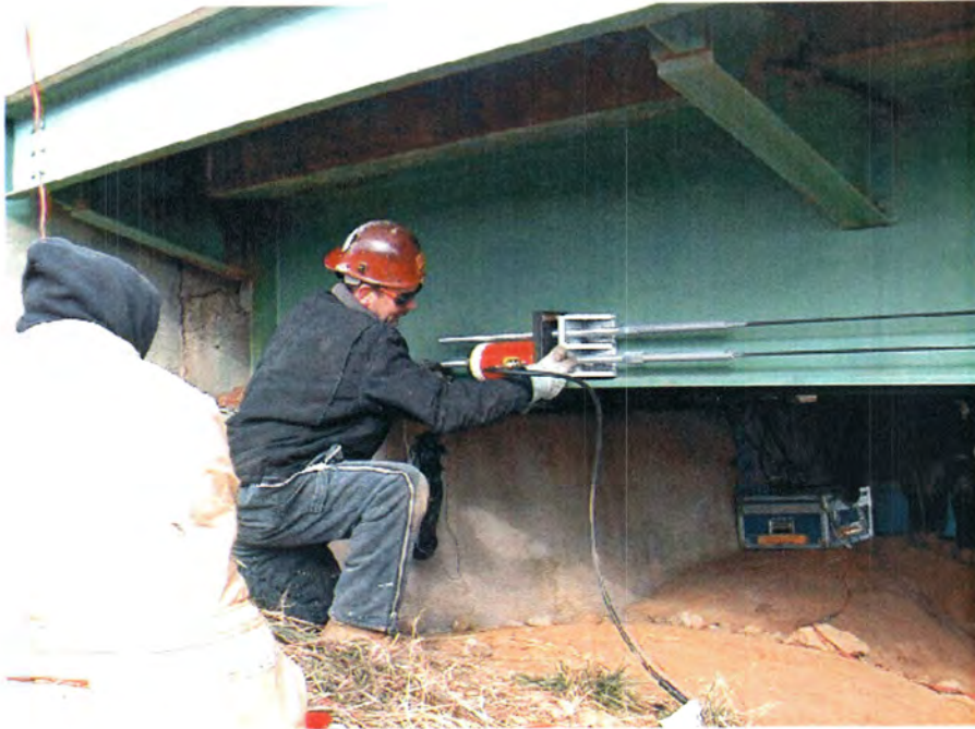
(a) Application of P-T force in the west end span
