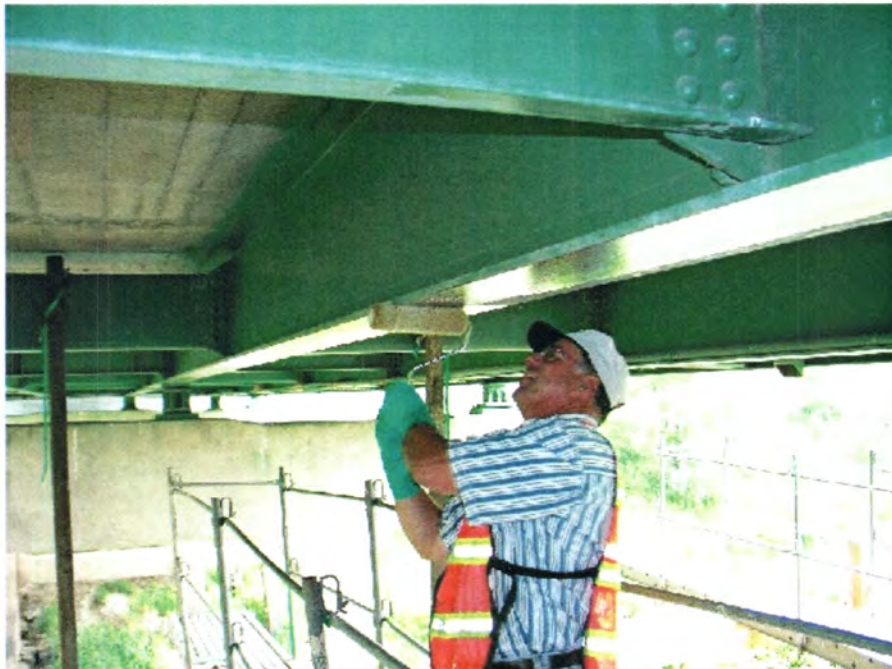
Figure II-14. Applying FRS 1000 Primer to bottom flange.
