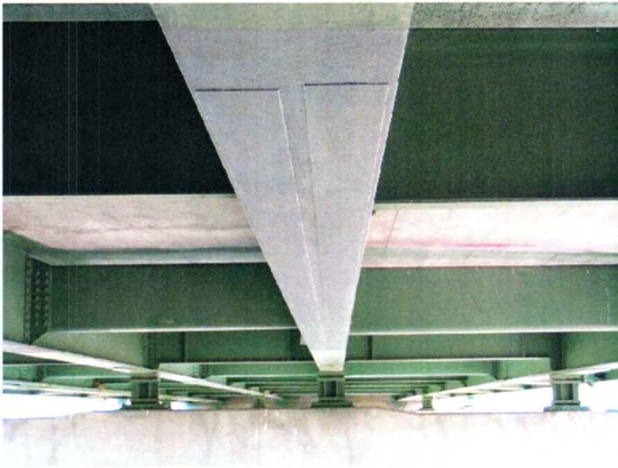
(b) Beam 3 in the west end span
