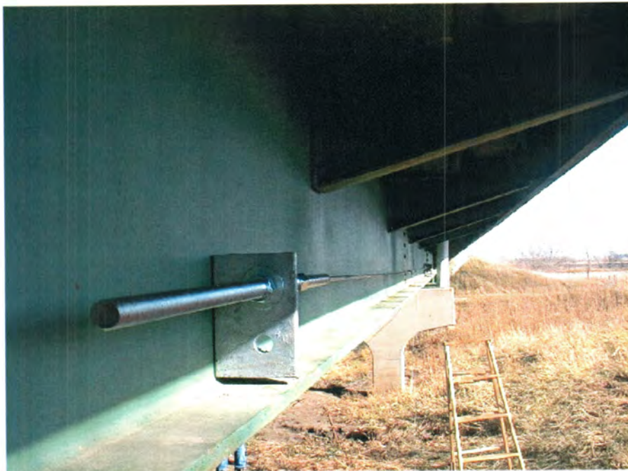
(b) Top CFRP bar in place
