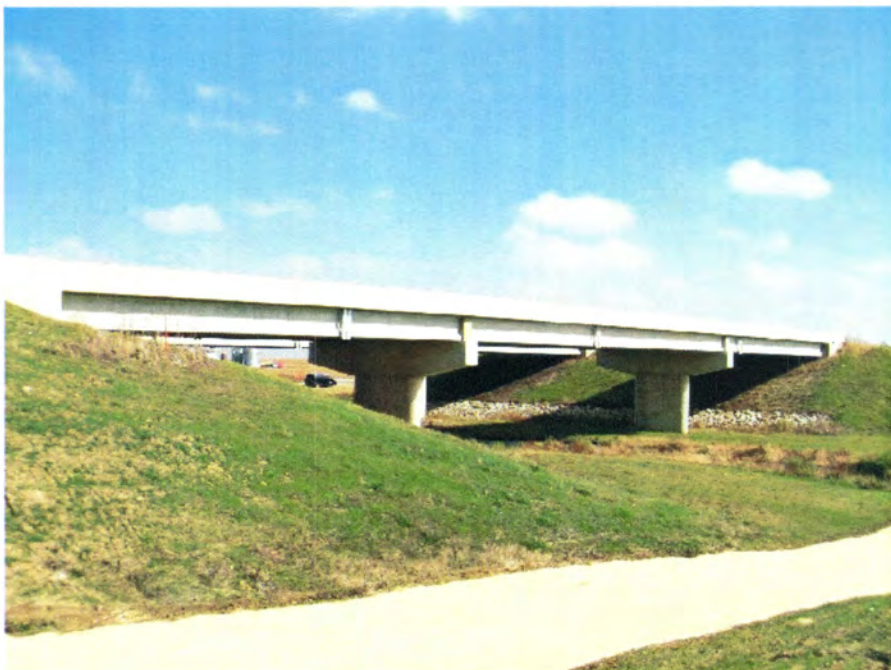
(a) Side view (MMFX bridge)
