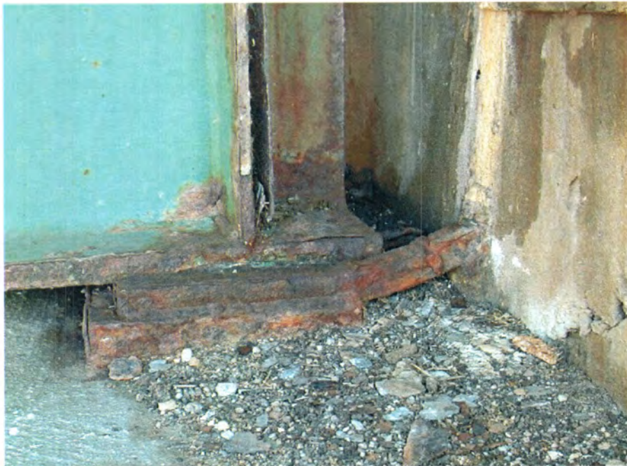
(d) Typical east abutment condition
