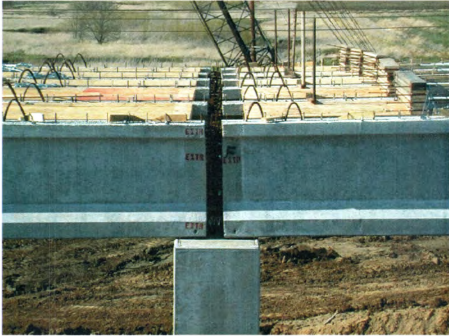
(c) Typical beam connection at pier
