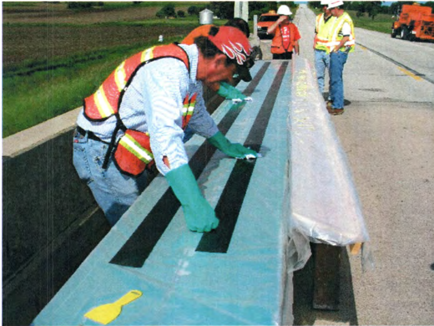
Figure II-13. Cleaning the CFRP plate bonding surface.
