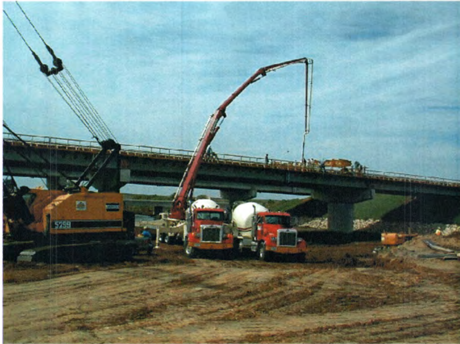
(c) Epoxy bridge (looking southwest)
