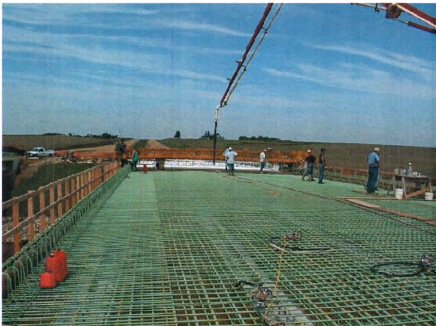
(d) Epoxy bridge (looking to the West)
