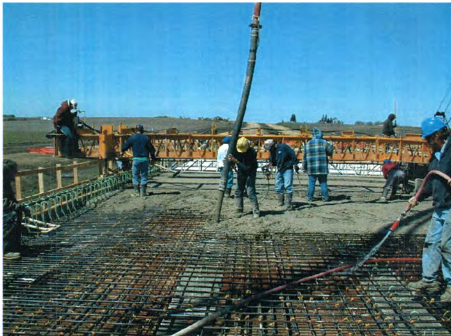
(b) MMFX bridge (looking west)
