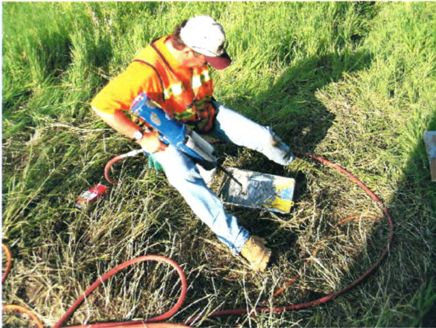
Figure II-15. Preparation of ECS 104 structural epoxy (mixing with a compressed air gun).
