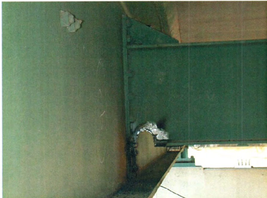
Figure I-6. Removal of a portion of the diaphragm/stiffener assembly.
