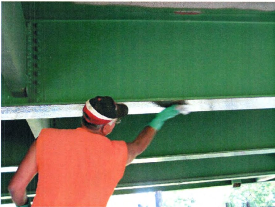
Figure II-12. Cleaning the beam surface after sandblasting.
