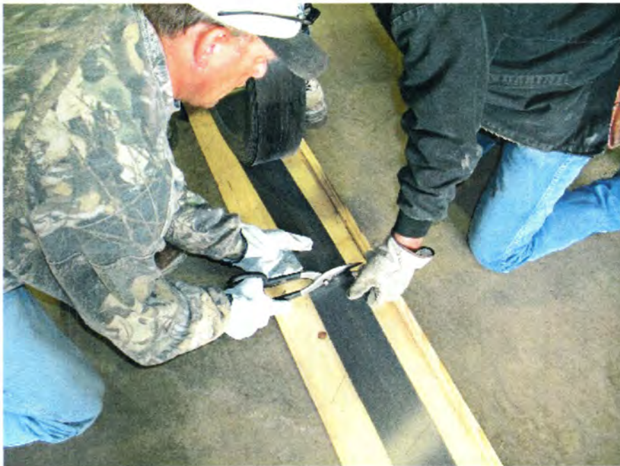
Figure II-16. Cutting the CFRP plates.
