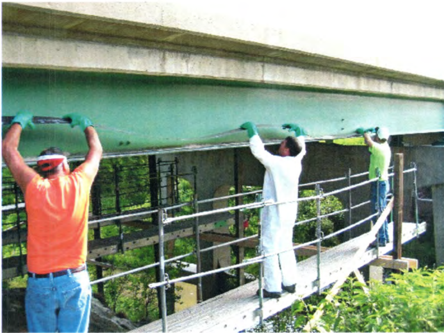
Figure II-18. Placement of CFRP plate on top of Beam 6 bottom flange.
