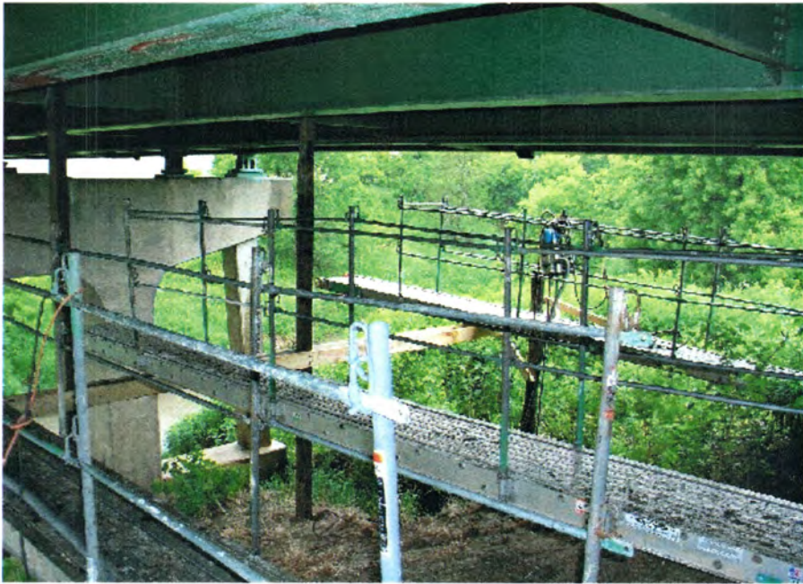
Figure II-9. Temporary work scaffolding.
