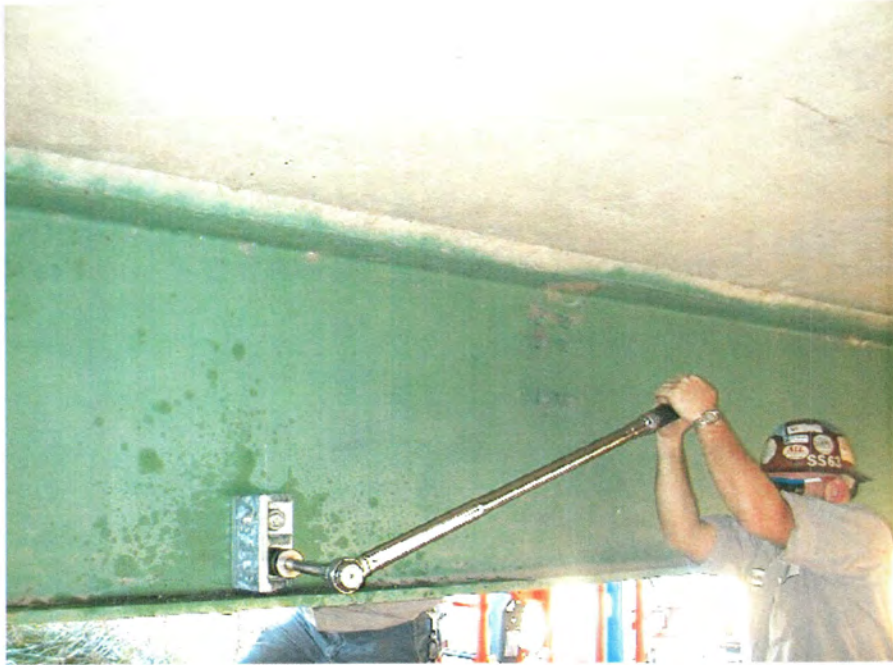
Figure I-5. Installing anchorage assembly.
