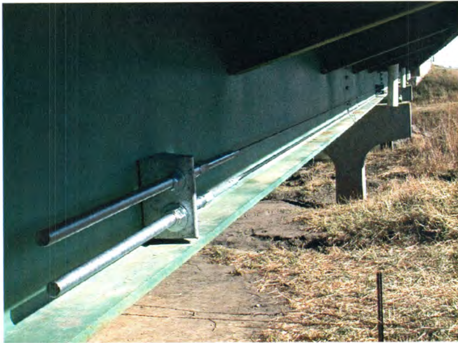
(a) Exterior CFRP bars in west end span
