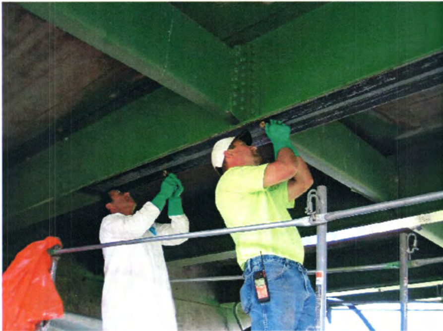
Figure II-19. Removal of excess air by applying pressure with a roller.
