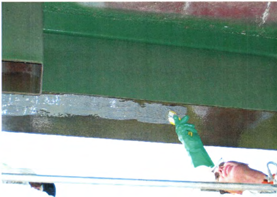
(b) Application of structural epoxy to bottom flange
